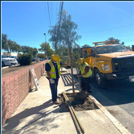
Cutting of new tree wells
