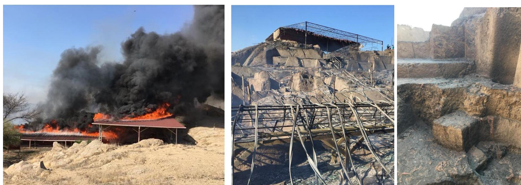
Fig.6 (Sx) Roof of the monument on fire (courtesy by Ignacio Alva); (medium and right) Damage caused by the fire (courtesy by Ignacio Alva)
